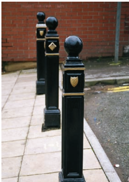
Bollards should only be used when absolutely necessary. Visual contrast will increase the visibility of these and other potential obstacles.
