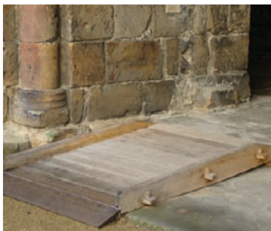
Removable timber ramps, such as this one at Richmond Castle in North Yorkshire, can provide access where a permanent intervention is not possible.
